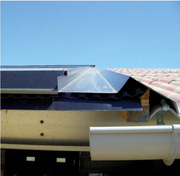
Lagerhalle, Dachanschlüsse
